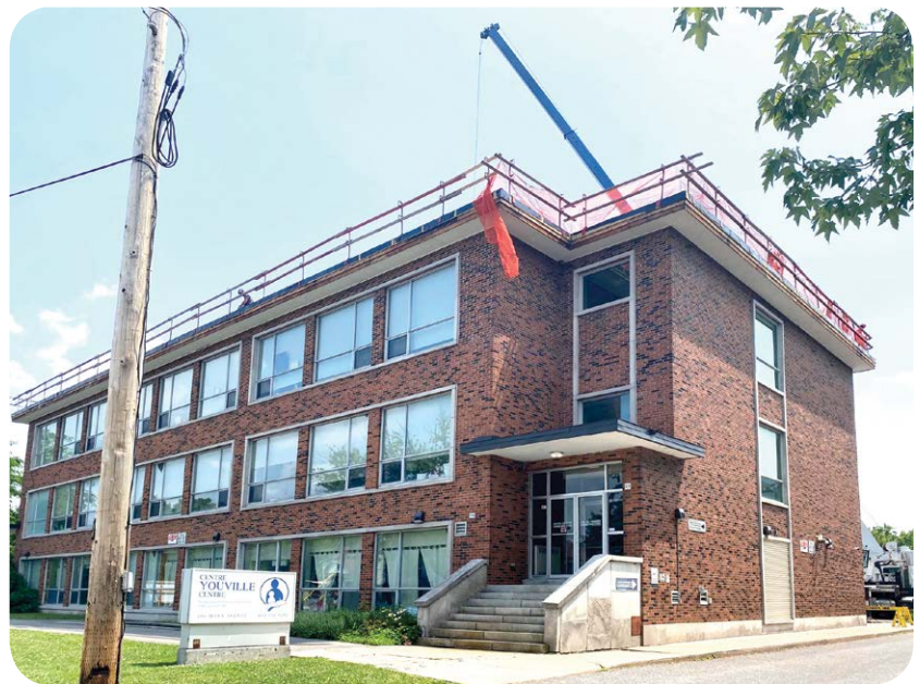
Photo of the building during construction with roof railings and a crane
